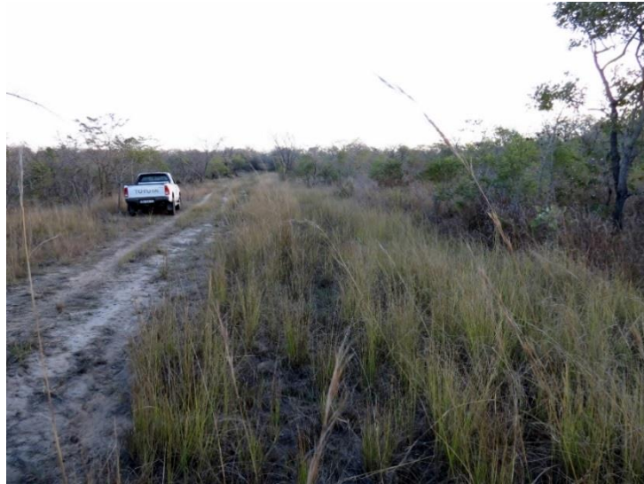
Clear signs of significant stormwater runoff in road
