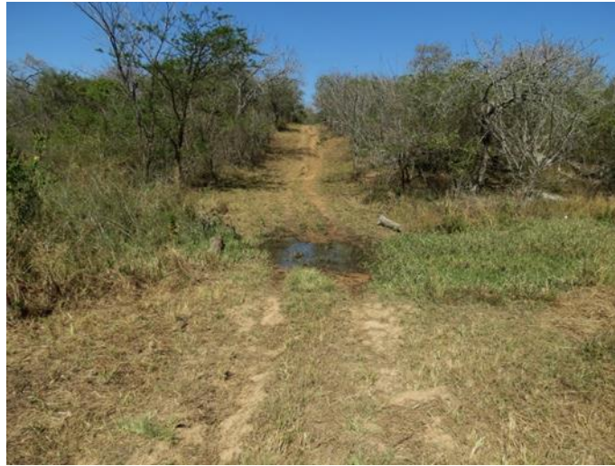
Typical road through wetland area
