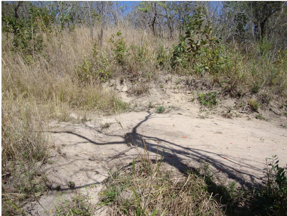
Figure 16: Earth structures (berms) and revegetate, intervention X31L-01-204-00
