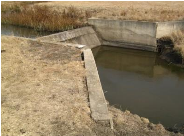
Figure 18: Earthen diversion berm, W42C-01-204-00 looking in a south-westerly direction
