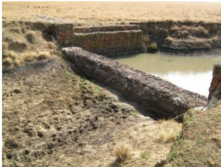
Figure 17: Intervention point C13C-04-202-00
