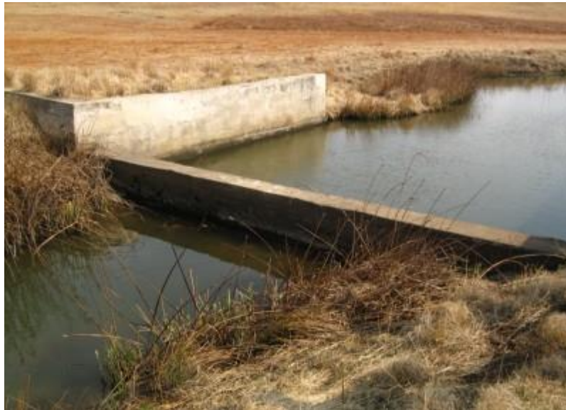
Figure 19: Intervention point C13C-04-204-00
