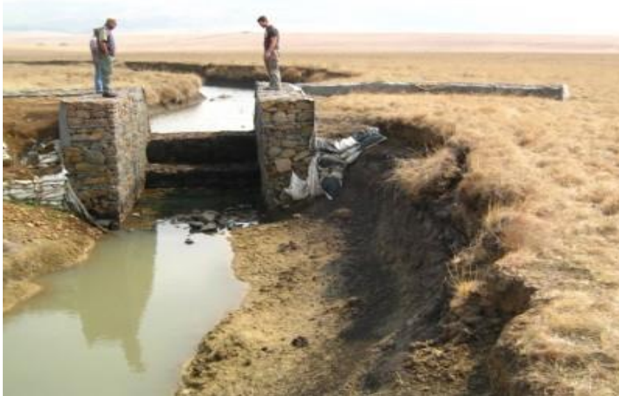
Figure 16: Intervention point C13C-04-201-00
