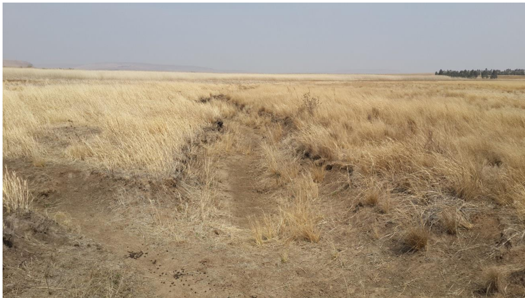
Figure 10: View SSE, looking upstream towards proposed intervention point (drop inlet) on the main eroded channel
