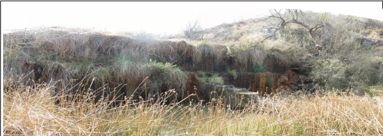
Dam wall in wetland area
