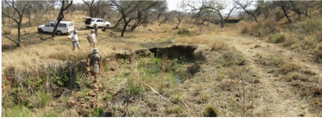
Earth Works, Rock Masonry schute with Gabion Road crossing (Capped)
