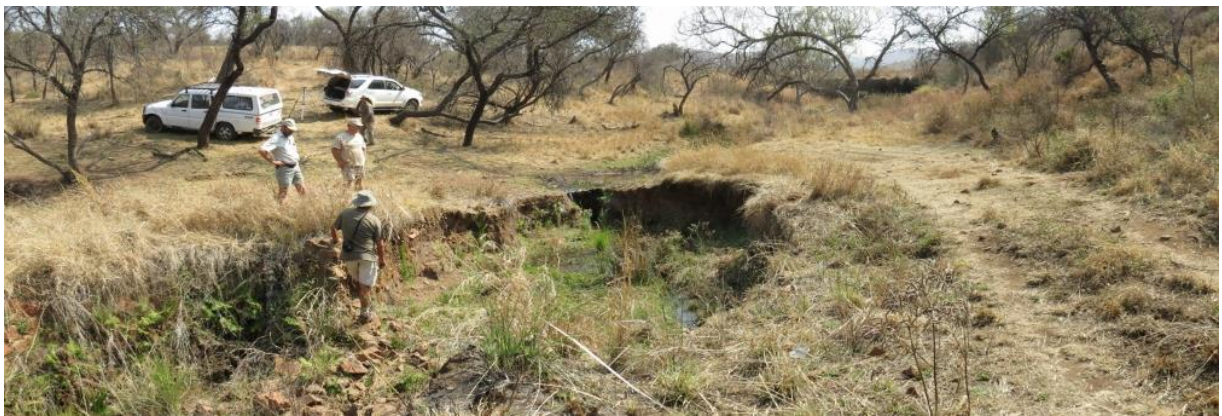
Figure 45: Headcut erosion with dam wall in background , B32A-02-201-01
