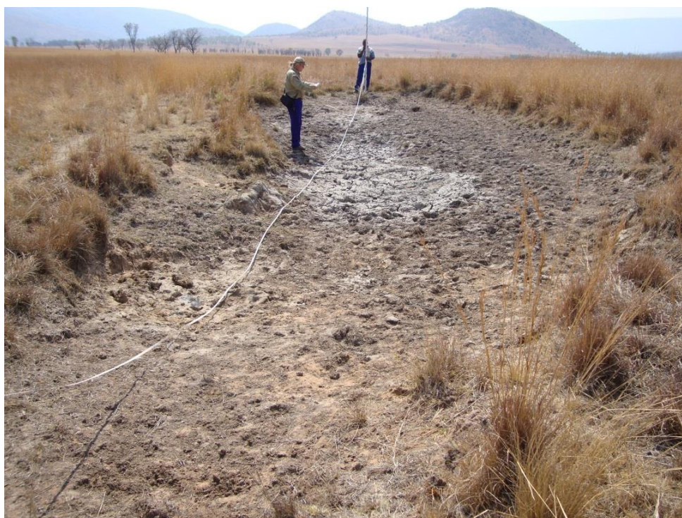
Figure 12: Rock packs with earth works, B32A-01-208-00
