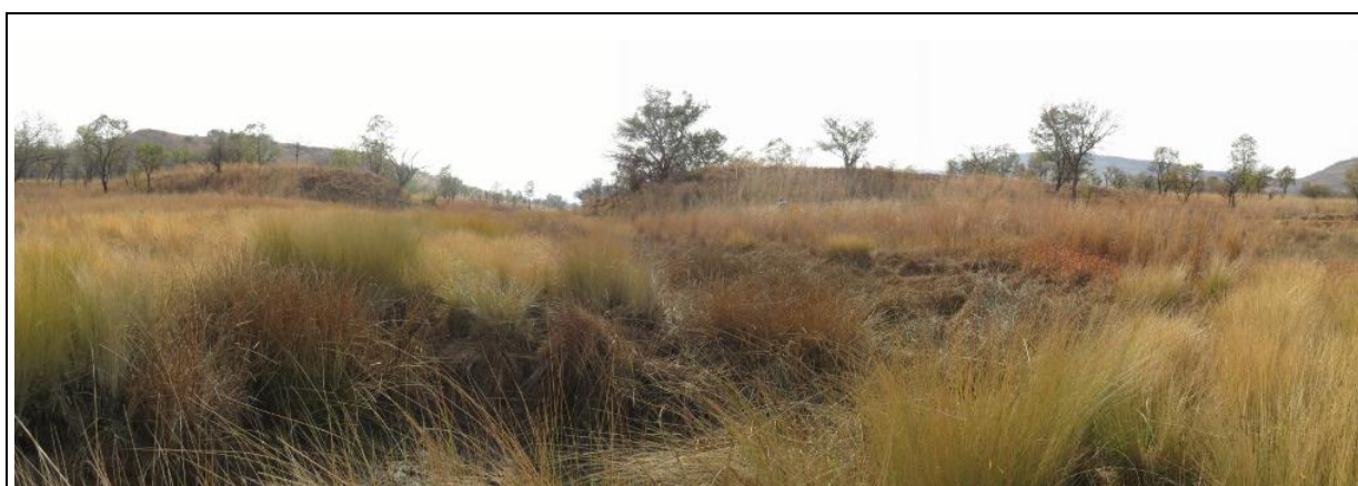
Broken dam wall in the back ground
