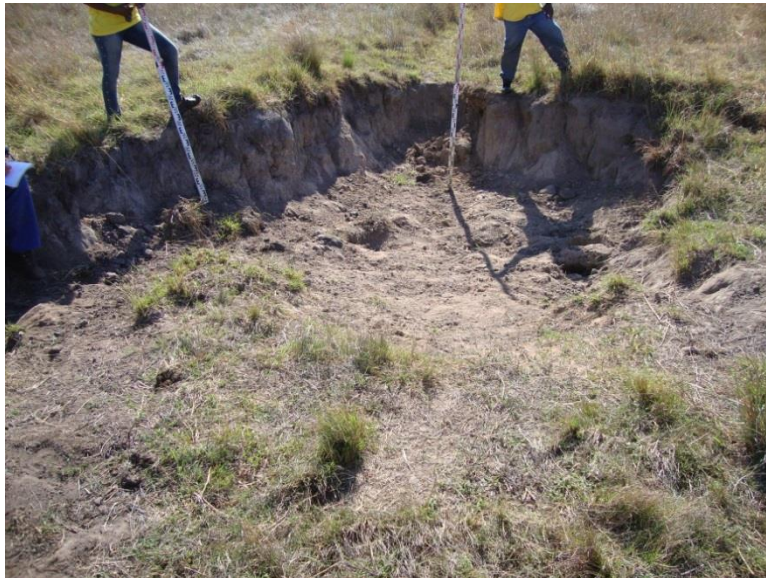
Figure 15: Intervention site A42D-01-250-00
