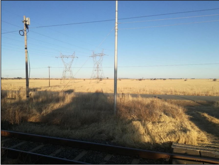
Figure 17: High voltage power lines in the study area
