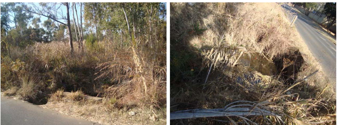
Figure 1: Drainage structures at Libertas Road
