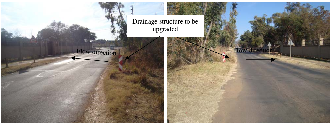
Figure 3 Libertas Road looking towards Stellenberg Road
