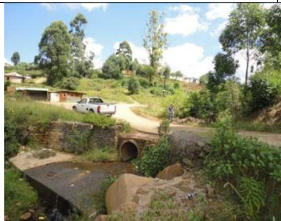
Figure 4: Main Watercourse crossing 2 looking north-west.
