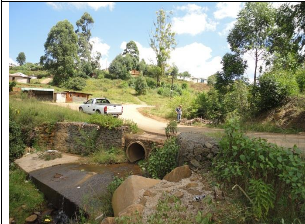
Figure 4: Main Watercourse crossing 2 looking north-west.
