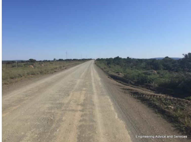
Figure 3 – Condition of Road MR00481
