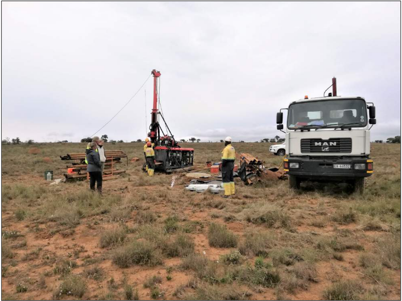
Plate 1: Rotary core drilling at borehole position E64
