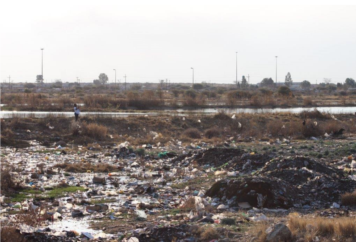
Photo plate 4.2: The Windsorton oxidation ponds and the Kutlong residential township in the background, Note evidence of sewage flowing into the landfill
