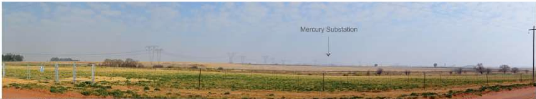
Photo 10b: View from the current grid line and the Mercury Substation.
