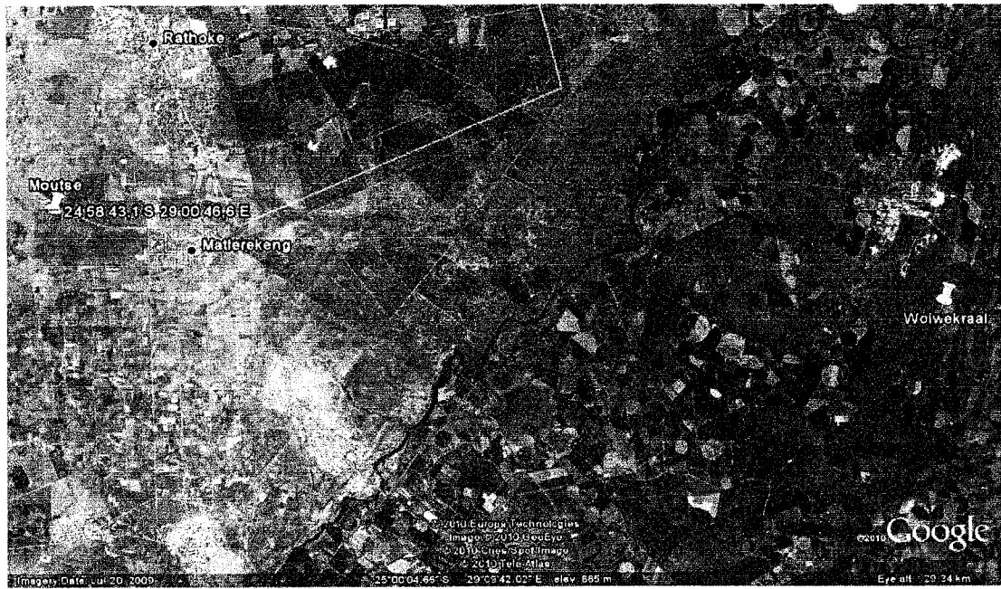
Figure 3 General view of the surveyed area between the Wolwekraal substation and the proposed Moutse substation. Note the disturbance by agricultural activities.
