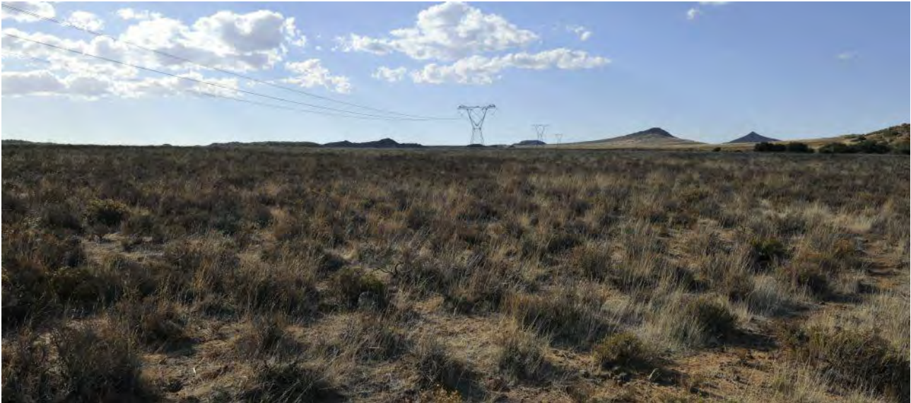
Figure 11: The Hydra-Poseidon 400kV 1 high voltage line running through the site.
