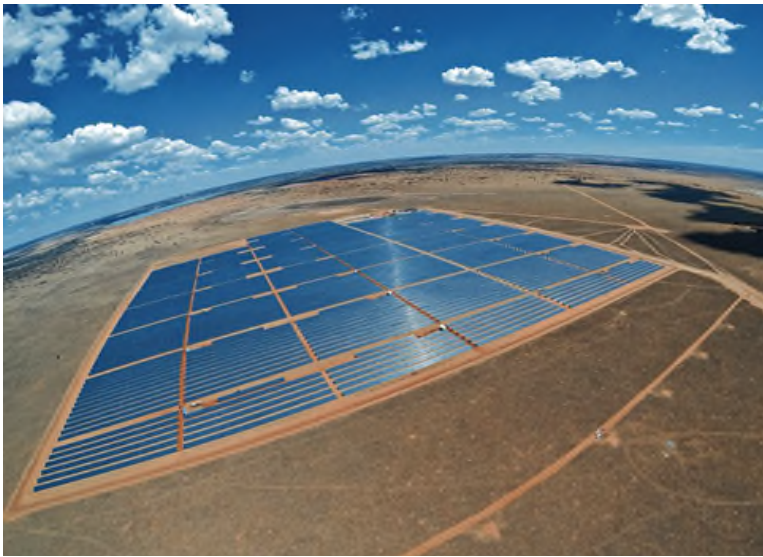
Figure 2.4: Photovoltaic (fixed-tilt/static) panel array (Photo: used with permission from Genesis Eco-energy Developments).
