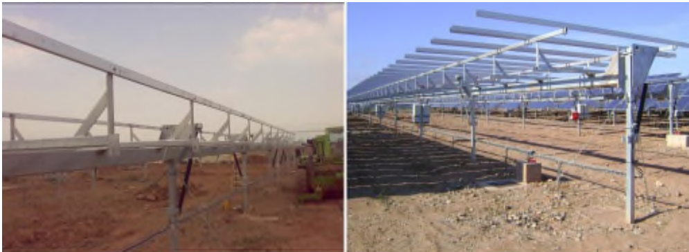
Figure 2.5: Frame, structural details (Photo courtesy of Igeam, 2011)
