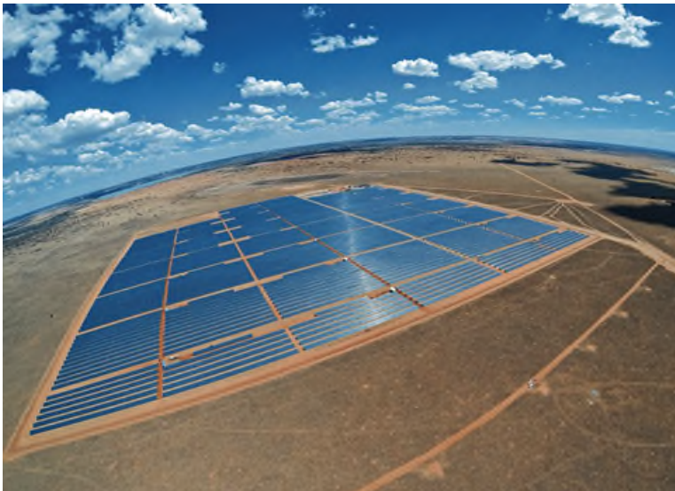
Figure 2.4: Photovoltaic (fixed-tilt/static) panel array (Photo: used with permission from Genesis Eco-energy Developments).
