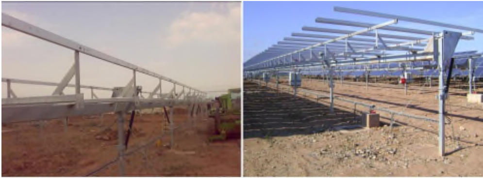
Figure 2.5: Frame, structural details (Photo courtesy of Igeam, 2011)
