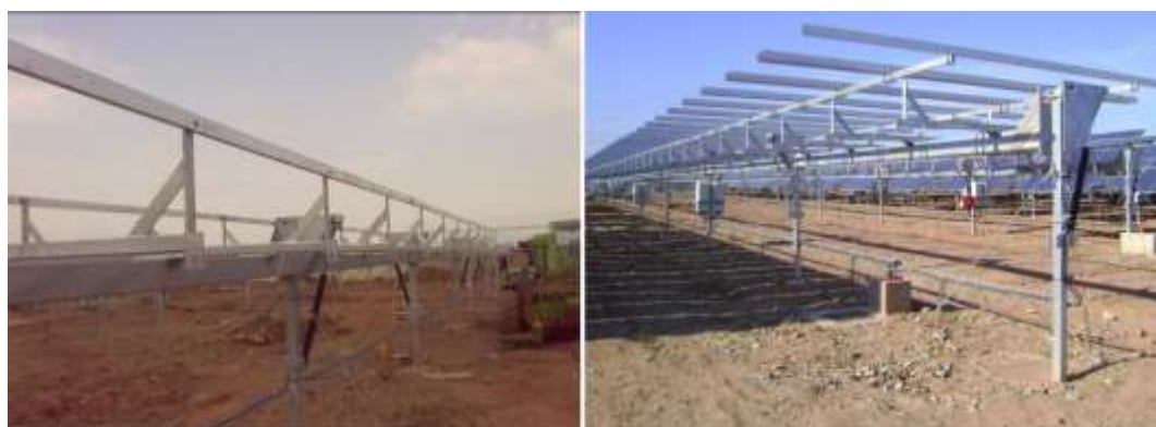
Figure 2.5: Frame, structural details (Photo courtesy of Igeam, 2011)
