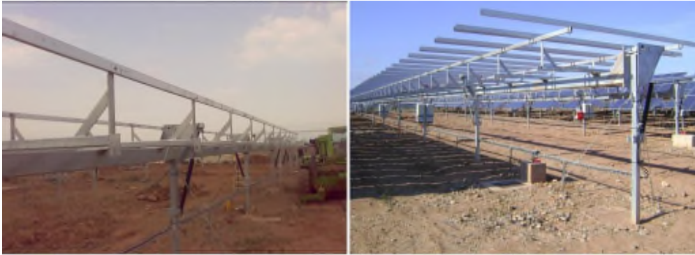
Figure 2.5: Frame, structural details (Photo courtesy of Igeam, 2011)
