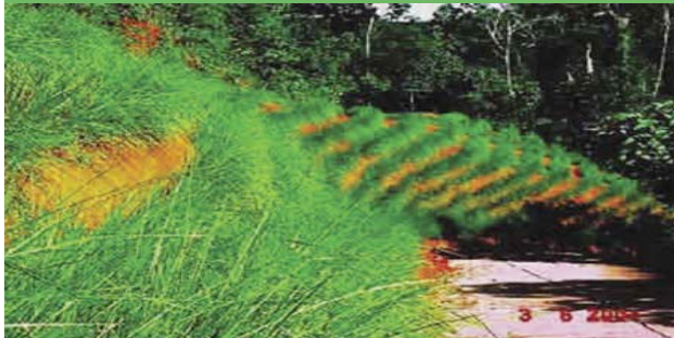
Venezuela - rehabilitation of bauxite mine tailings. The soils are very acid and prone to slippage. High levels of fertilizer assure good growth
