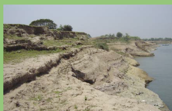
Cambodia - This very large bank on the Mekong River has been under continuous erosion. The land owner with assistance from TVNI is stabilizing using vetiver hedgerows.
