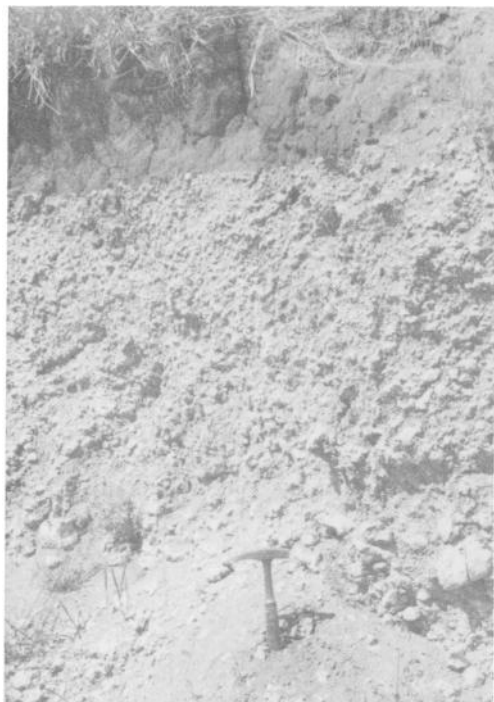
FIG. 4. Nodular calcrete (Netterberg 1980). Calcrete cobble in lower right hand corner is a weathering relic of an older hardpan calcrete and not a nodule.
