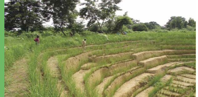
Congo D.R. - huge gullies that destroy urban areas and houses can be rehabilitated and stabilized using the Vetiver System.
