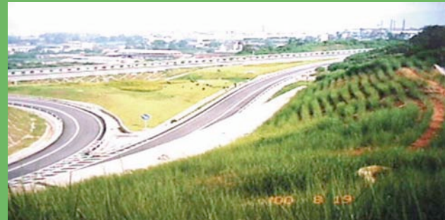
China - expressway stabilization. This cut was prone to massive slip. Stabilization with VS has given complete protection
