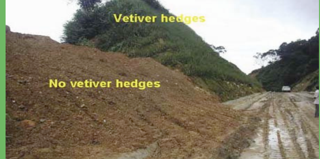
Vietnam - Ho Chi Minh Highway - with and without vetiver stabilization
