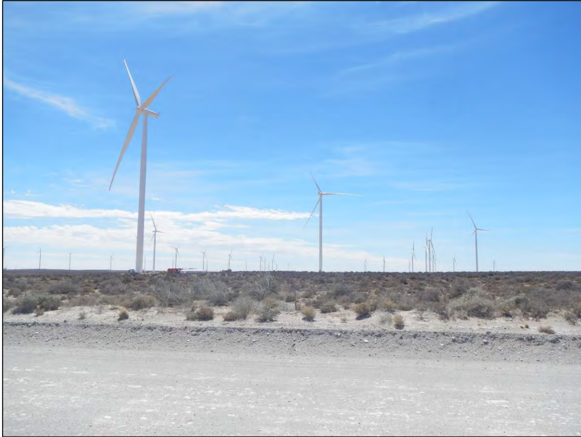
Figure 20: View of the Loeriesfontein Wind Farm which has been constructed approximately 29km to the east of the proposed Xha! Boom Wind Farm application site. This wind farm is however located outside of the visual assessment zone and is therefore not expected to alter the visual character of the study area.
