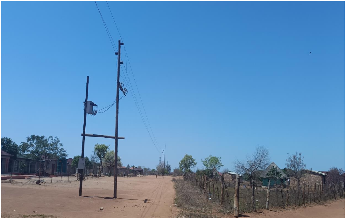
Shows the existing powerline on site
