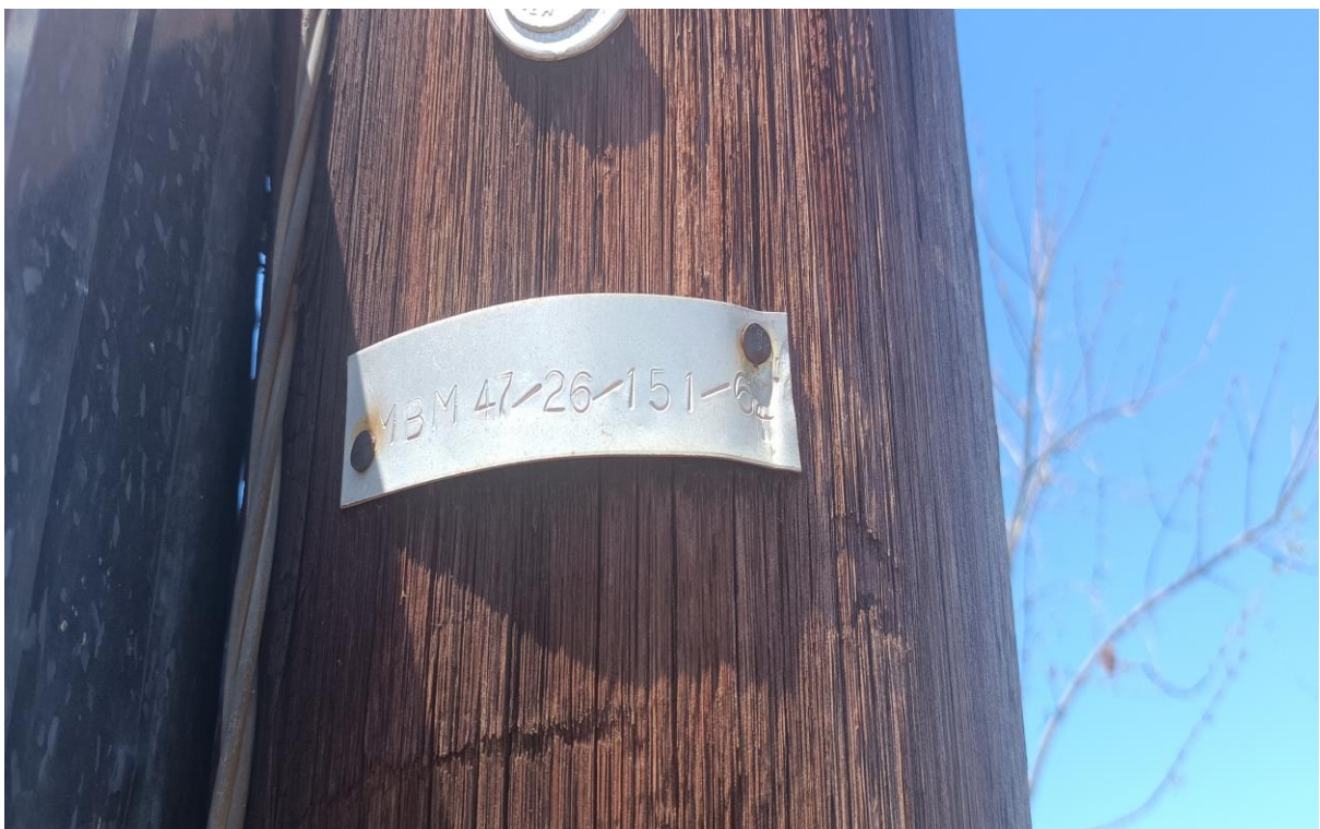
Shows the existing pole number
