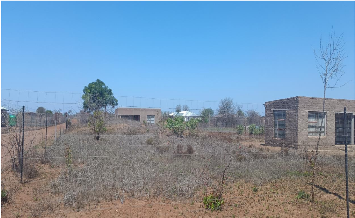
Shows the area where electricity is required
