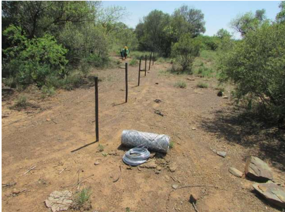
Figure 2: Erecting the fence around Site 12.
