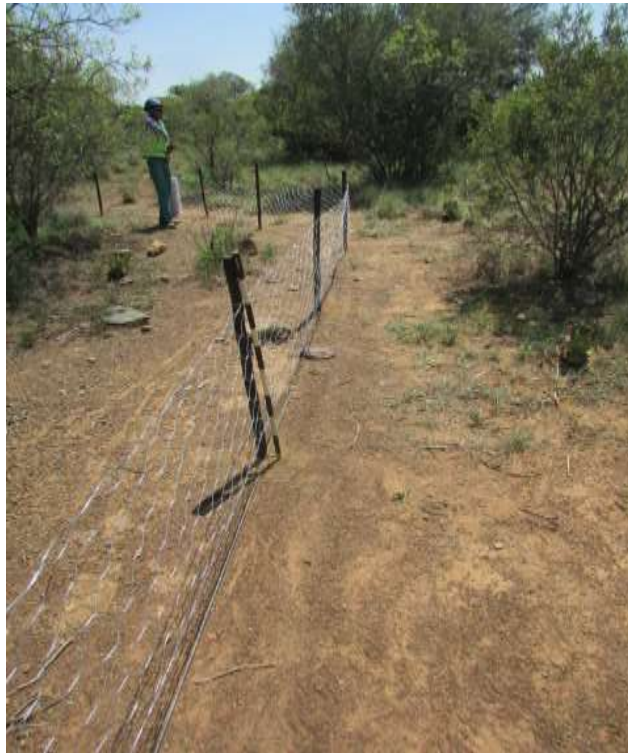
Figure 3: The fencing around Site 12 nearing completion.
