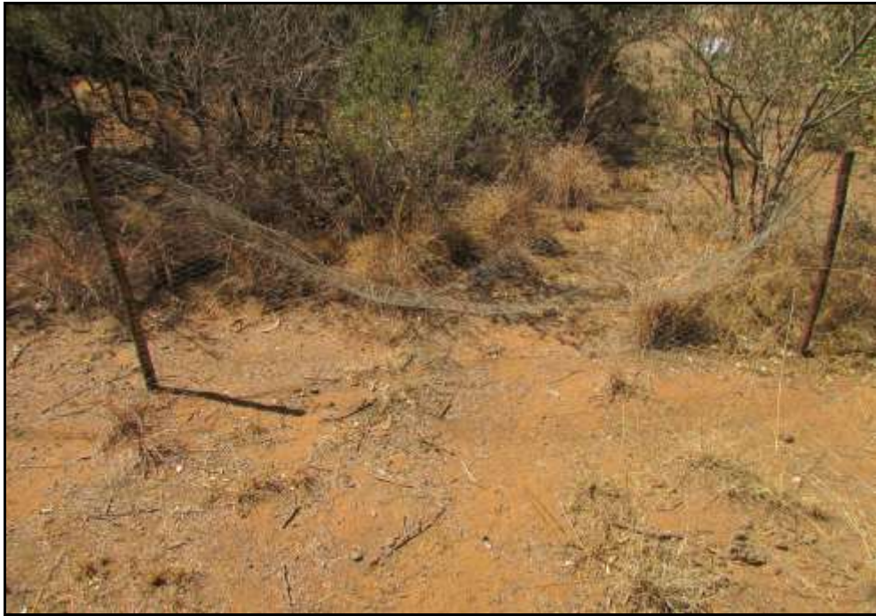
Figure 33: A section of fencing around Site 12 that had been broken and needed to be fixed.
