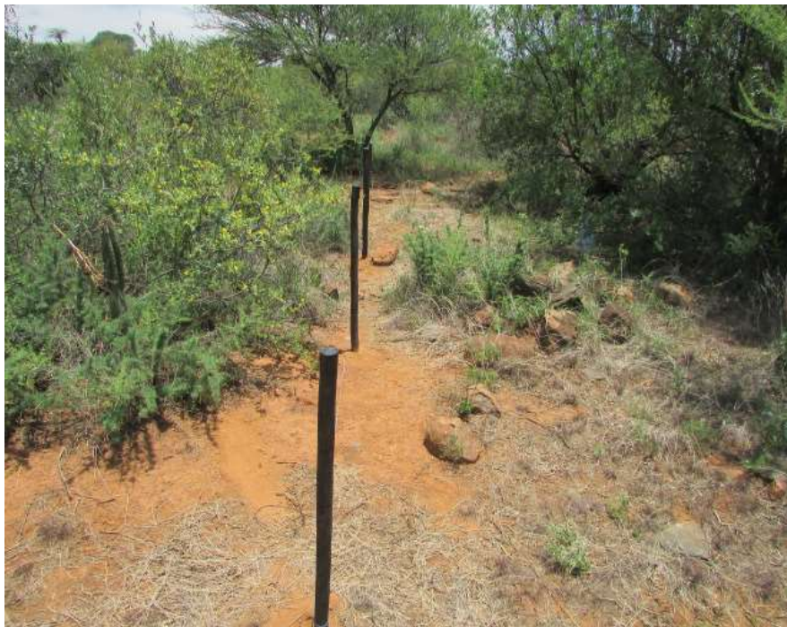
Figure 5: Fencing at the New Site in progress.
