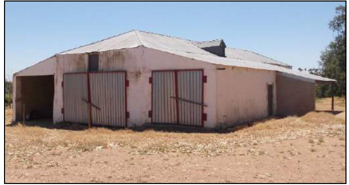
Figure 31: The outbuilding/barn at Die Mond.
