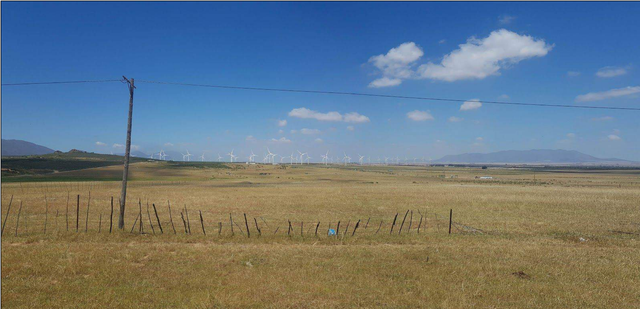
Figure 7.3b. Photograph Simulation. From Point 5 - Road towards Saron - as per EA (110m hub height)
