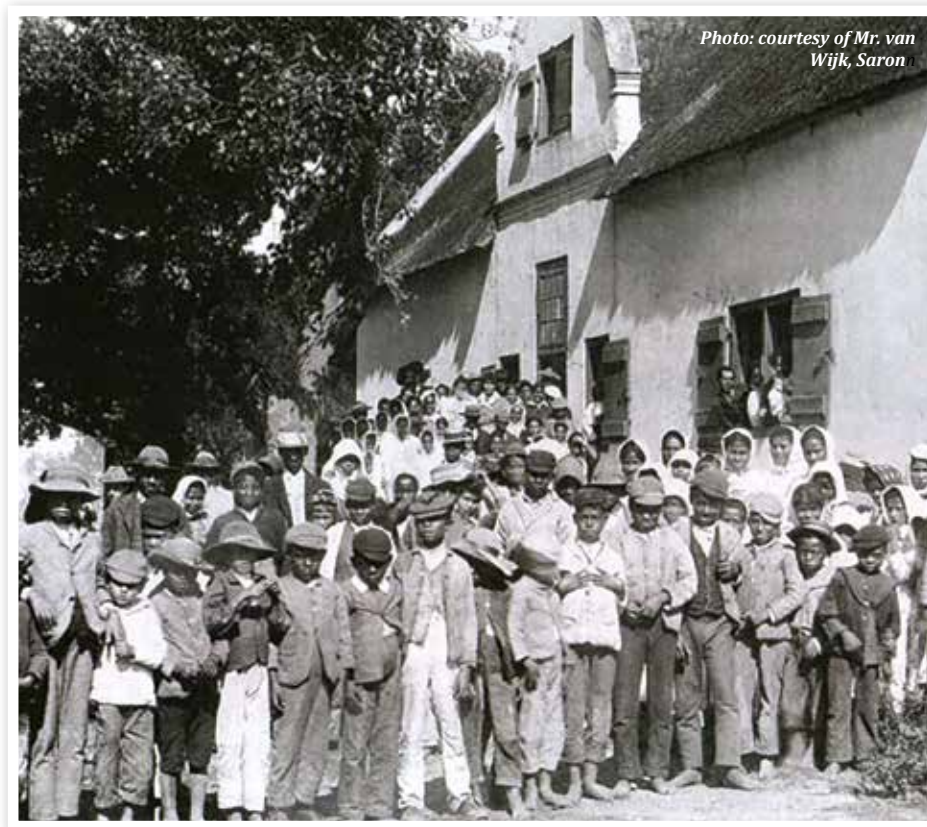
FIG 3A A rare historical photograph of the De Leeuwenklip homestead (and group of mission children) when it was still largely intact (c.1910). Note the thatched roof, double casement windows with shutters, and fanlight (now all gone). A modern facebrick veranda added a few decades ago has now obscured most of the facade, which has also been given sash windows and a French front door.
