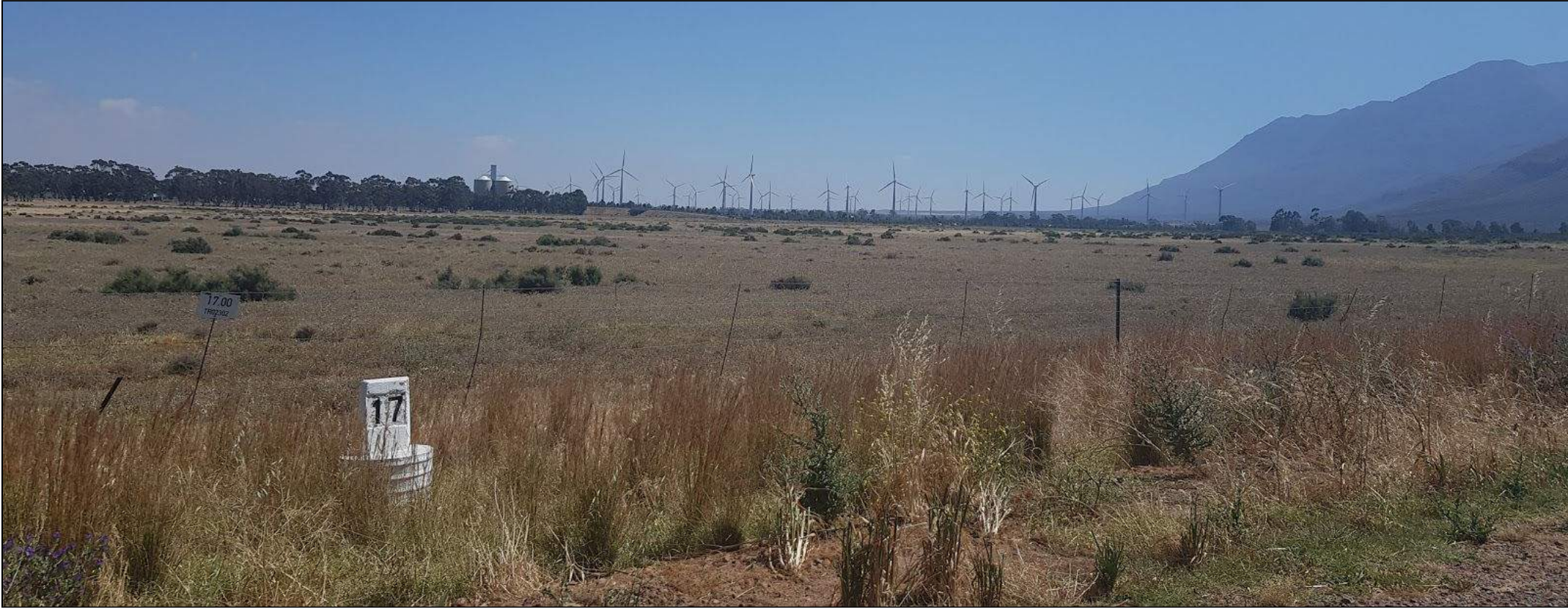
Figure 6.1. Contextual Photographs. October 2019, Existing turbines of the Gouda WEF
