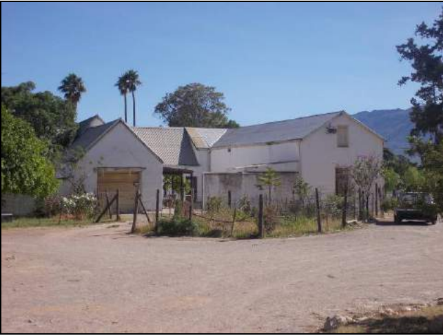
Figure 35: The rear of the parsonage.
