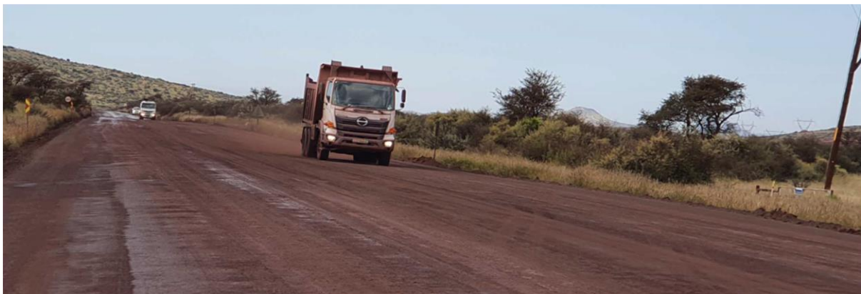
Figure 10-15: Dust Suppression on the DR03333 Provincial Road
