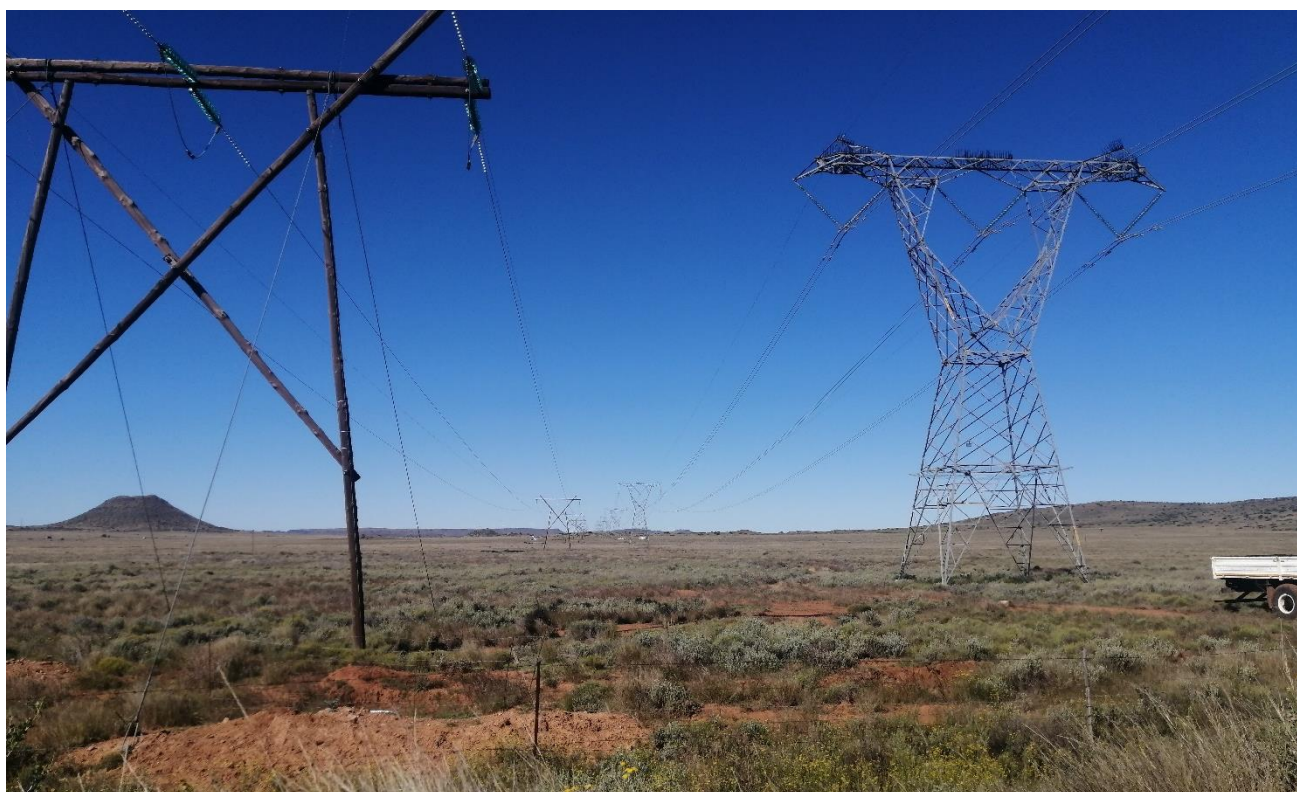
Figure 10: Electrical infrastructure that traverses the study area
