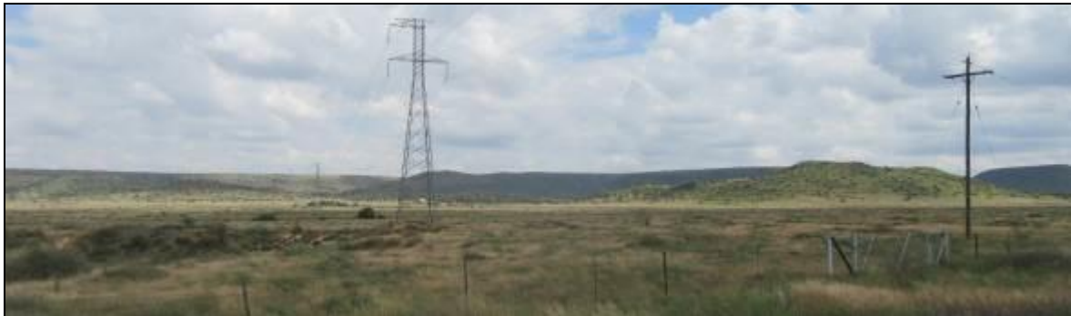
Photograph 3.4: Transmission line on Ruspoort
