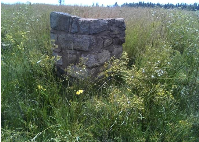
Figure 2.10: Feature 1 - Stone and cement wall.
