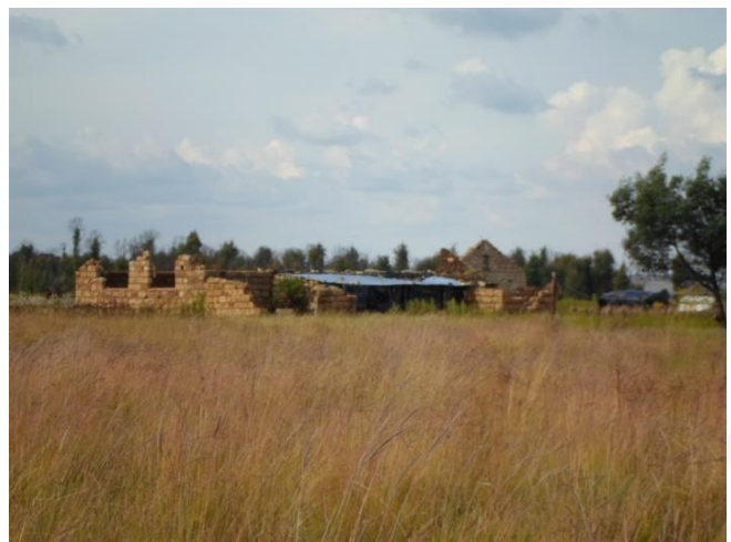
Figure 2.13: Partially demolished sand stone structures.
