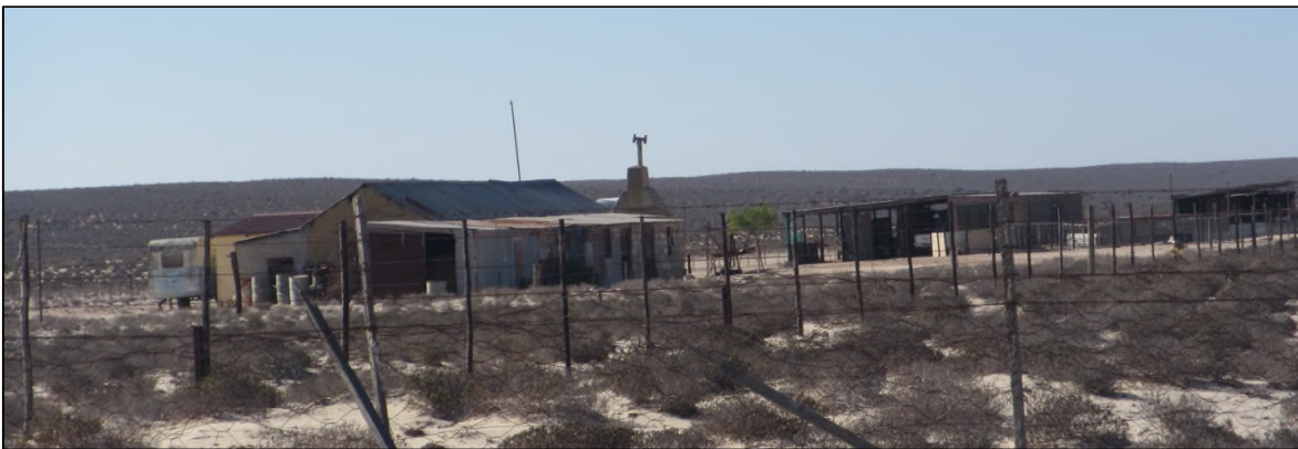
Figure 17: View of the outbuildings at Zonnekwa 326 as seen from the southeast.
