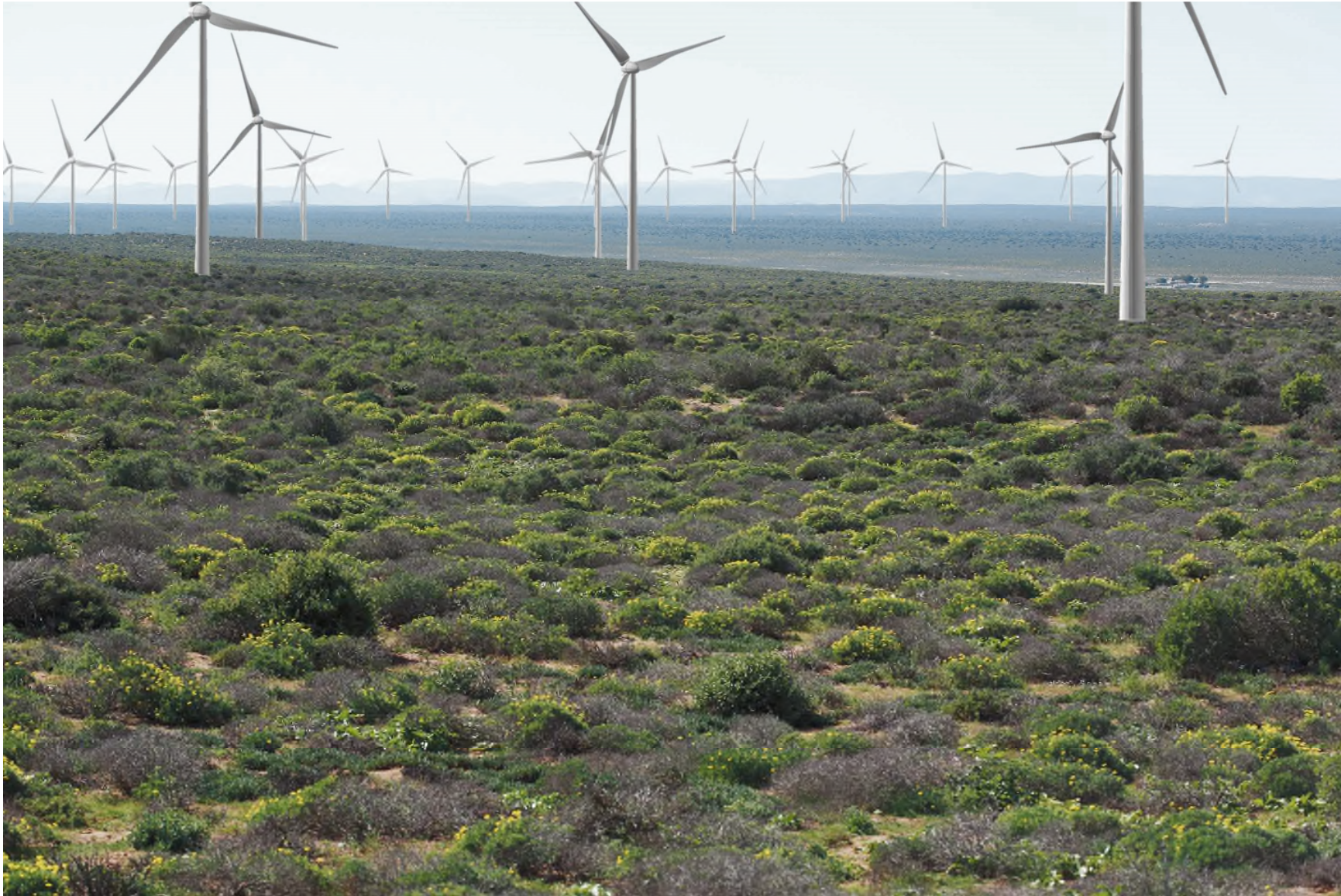
Figure 17: Photo simulation 4 (after construction).
