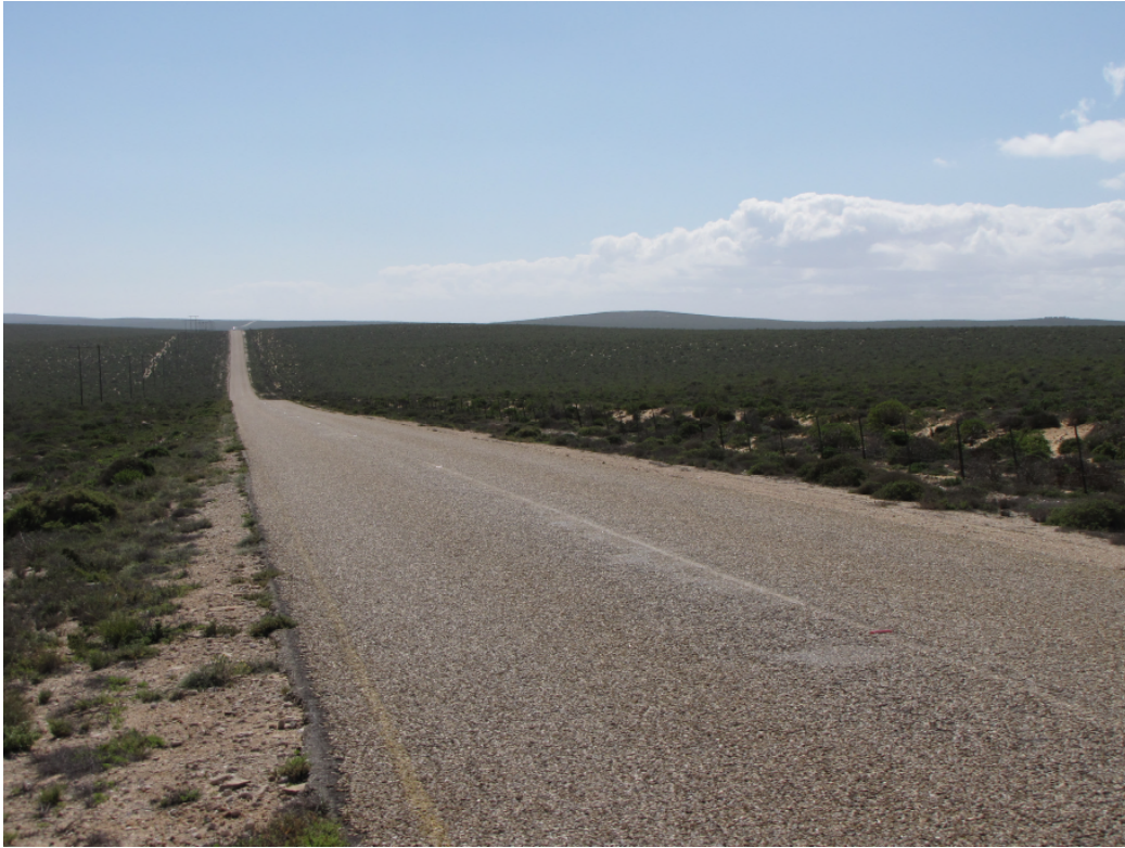
Figure 3: The Koingnaas to Kleinsee road west of the proposed project site.
