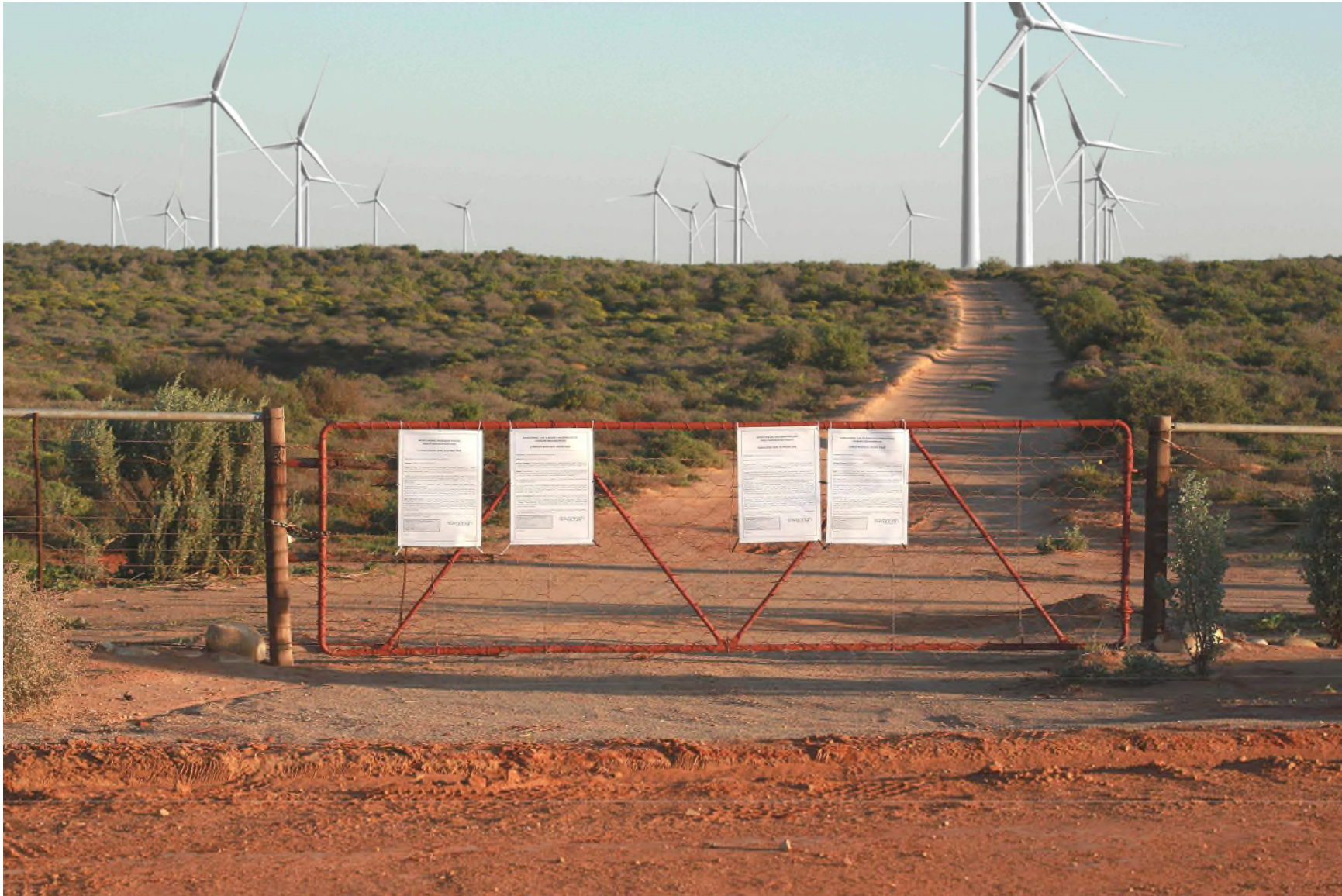
Figure 13: Photo simulation 2 (after construction).
