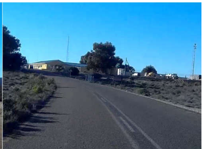
Photograph 2-12: MR751 Surfaced Section
