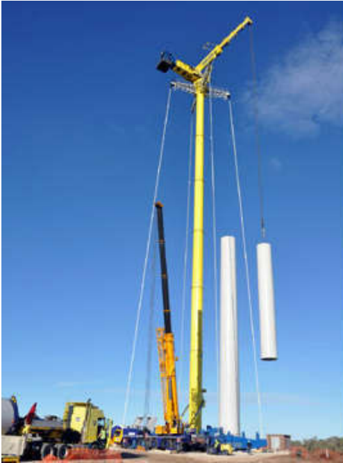
Figure 3-6: Cranes at work (Source: Author's photograph)
