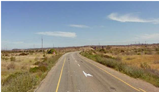
Photograph 2-1: Saldanha Bay Rd
