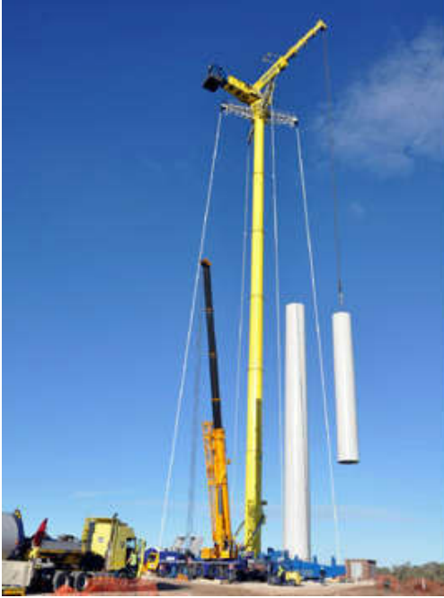
Figure 3-6: Cranes at work (Source: Author's photograph)
