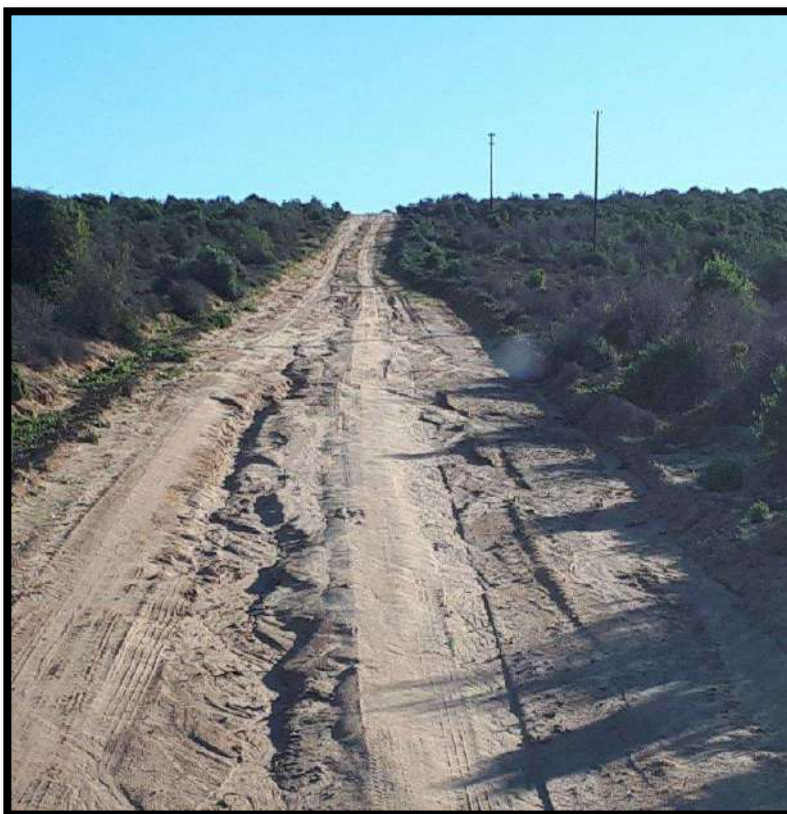
Figure 1-8: Note the erosion damage along the main farm access roads with sandy soil condition, running on relative steep gradients.
