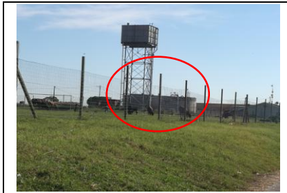
Photo 1A: The Shongweni Reservoir (Photographer facing North West)
