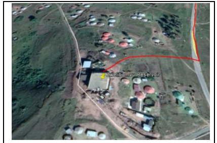
Photo 1B: The Zwelibomvu 2 Reservoir (Google Earth, 2019).
