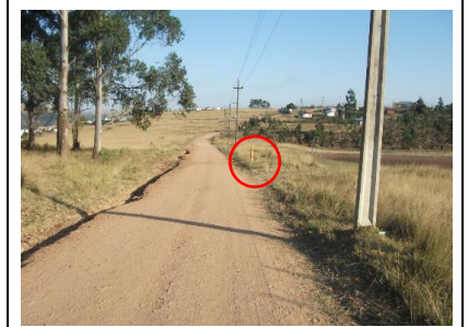
Photo 1C: Existing pipeline (in red) located within the road reserve, alongside multiple power lines (JLB Consulting, 2019).
