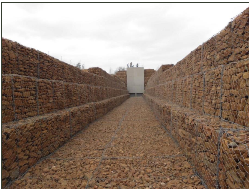
Figure 8 Example of a gabion channel (Vaal River abstraction, Aurecon project)
