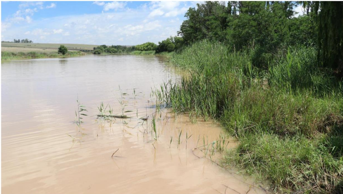
Figure 8: The weir clearly results in an elevation of the baseflow level of the river. The banks would naturally have been much broader and more diverse in terms of habitat and geomorphology.
