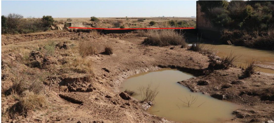
Figure 12: Upstream of the weir (red), sediment accumulation is evidently quite high and this will certainly affect the flow, flooding and sediment regime of the river, at least at the site.
