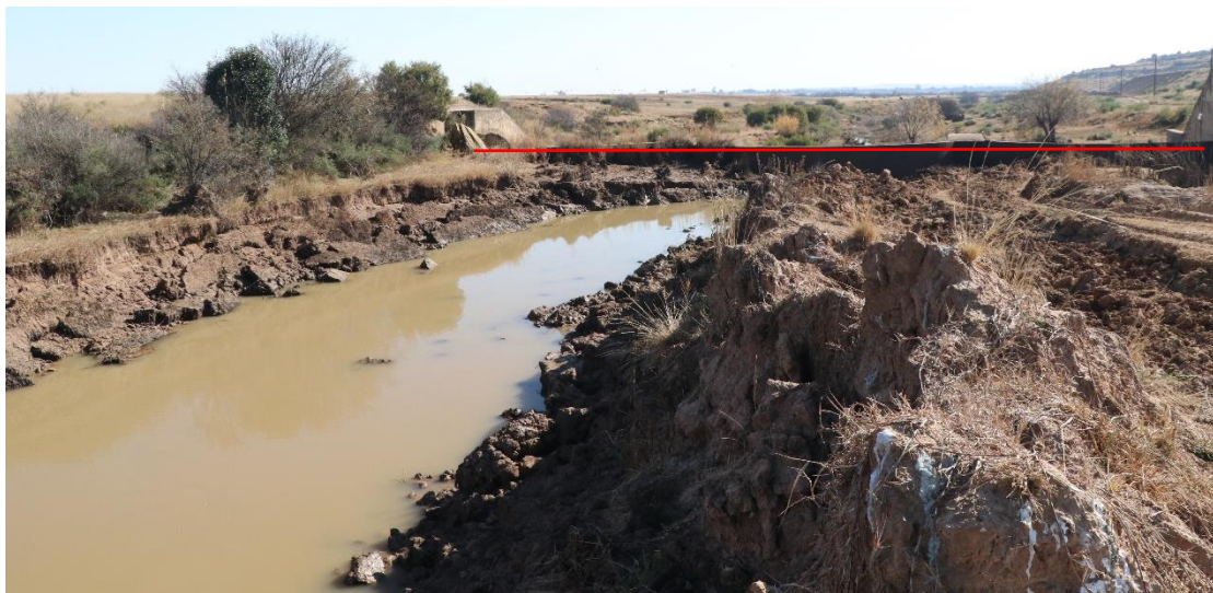
Figure 3: View of the weir (red) at the site. Extensive sediment deposition is visible in the foreground.
