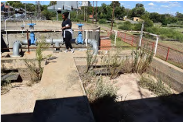
Figure 3 | Filters (with exposed aggregate and weeds)
