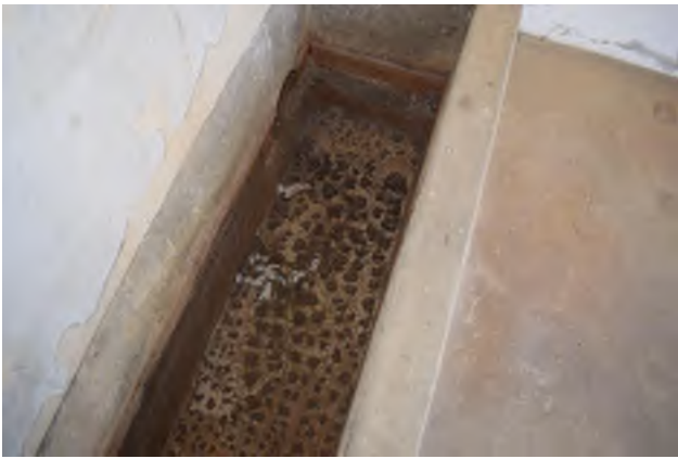
Figure 1 | Exposed aggregate in inlet channel
