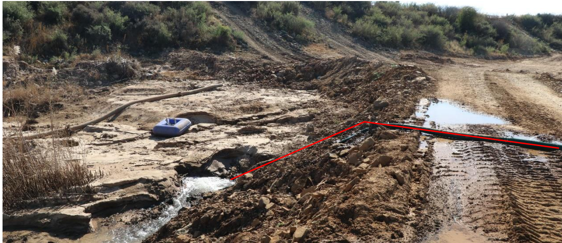
Figure 16: The construction activities also entail dewatering of construction areas which contain sediment loads.
