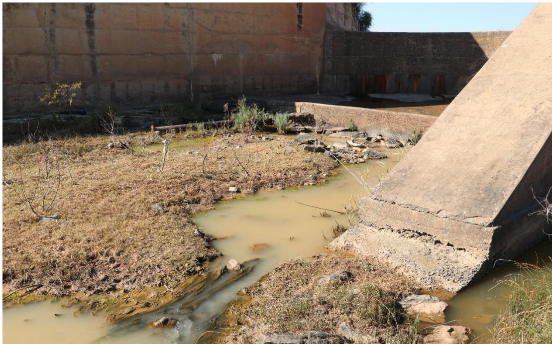
Figure 17: Water released from the construction area into the river clearly contains a sediment load which will also have an impact on the river. This should also provide an indication of the anticipated impacts that dredging will have.
