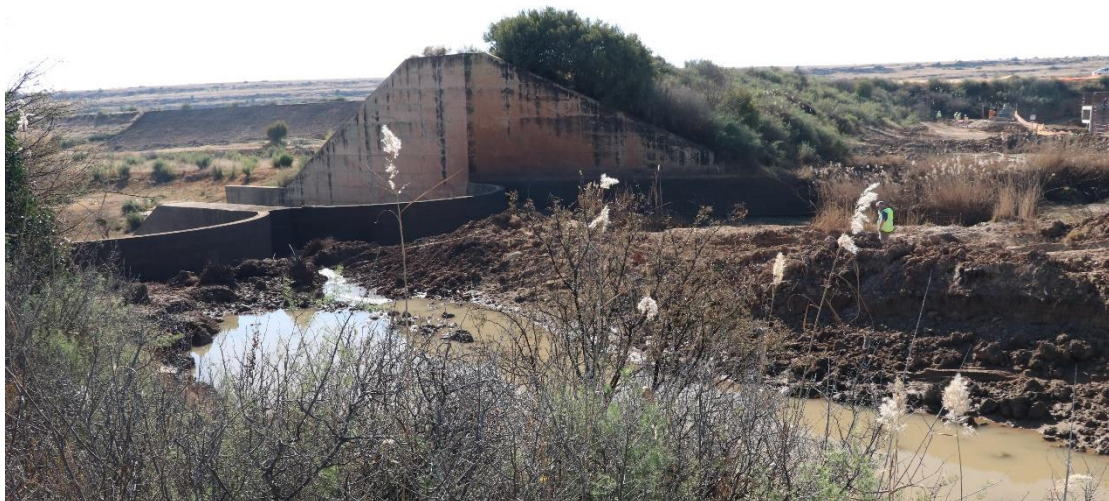
Figure 13: Upstream of the weir the river has a shallow main channel with high volumes of sediment being evident.
