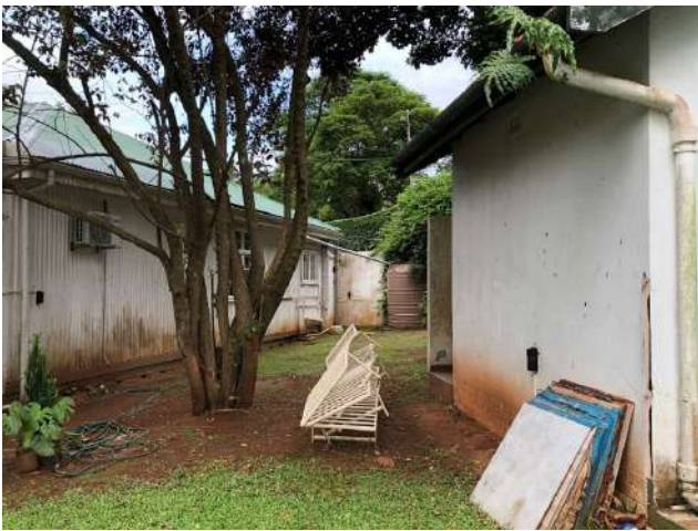
Image 3 – Above of Out building & Main Dwelling
