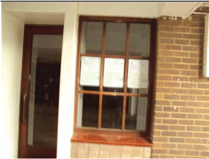
Photo 11 Site Notice Placement - Mkhondo Municipality
