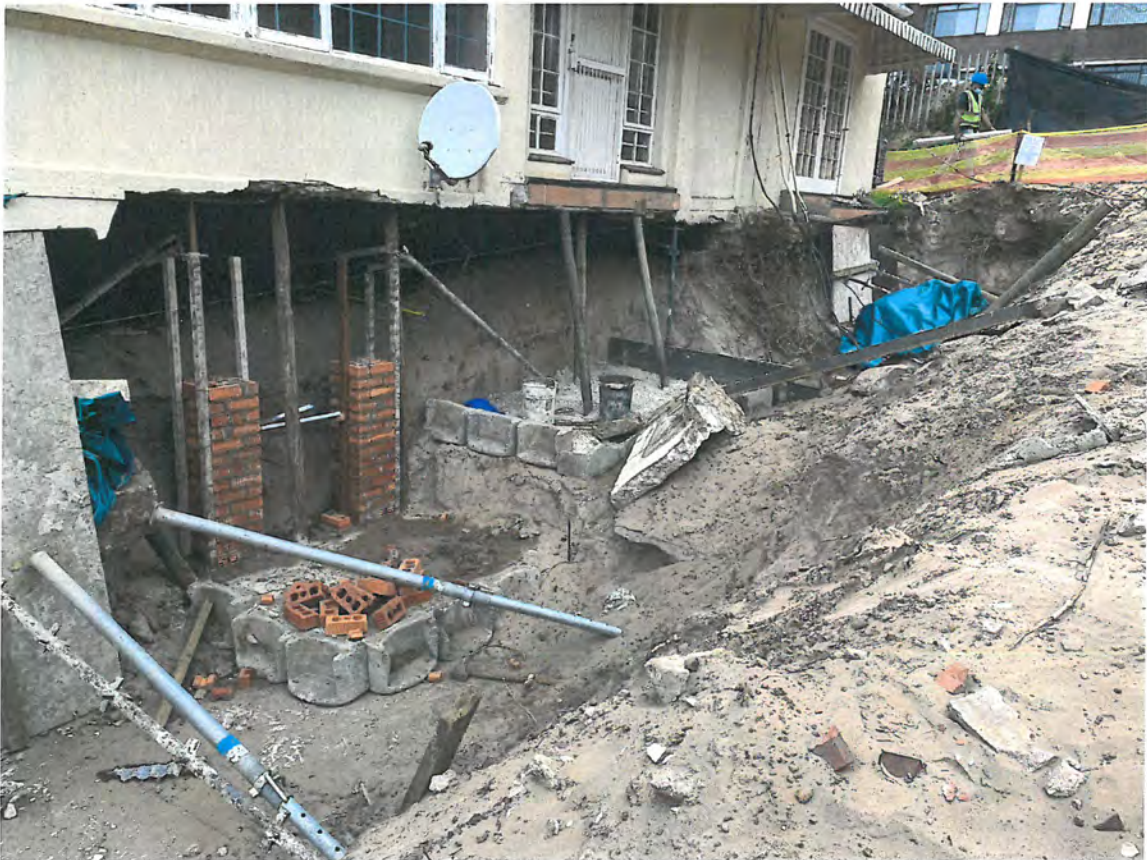
Emergency propping and repairs in progress 17 November 2021
