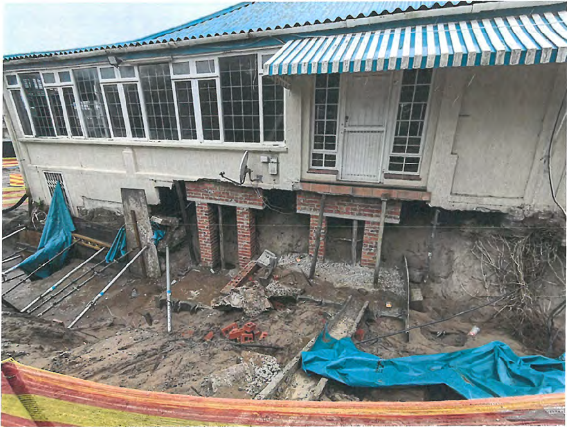
Emergency propping and repairs in progress 25 November 2021
