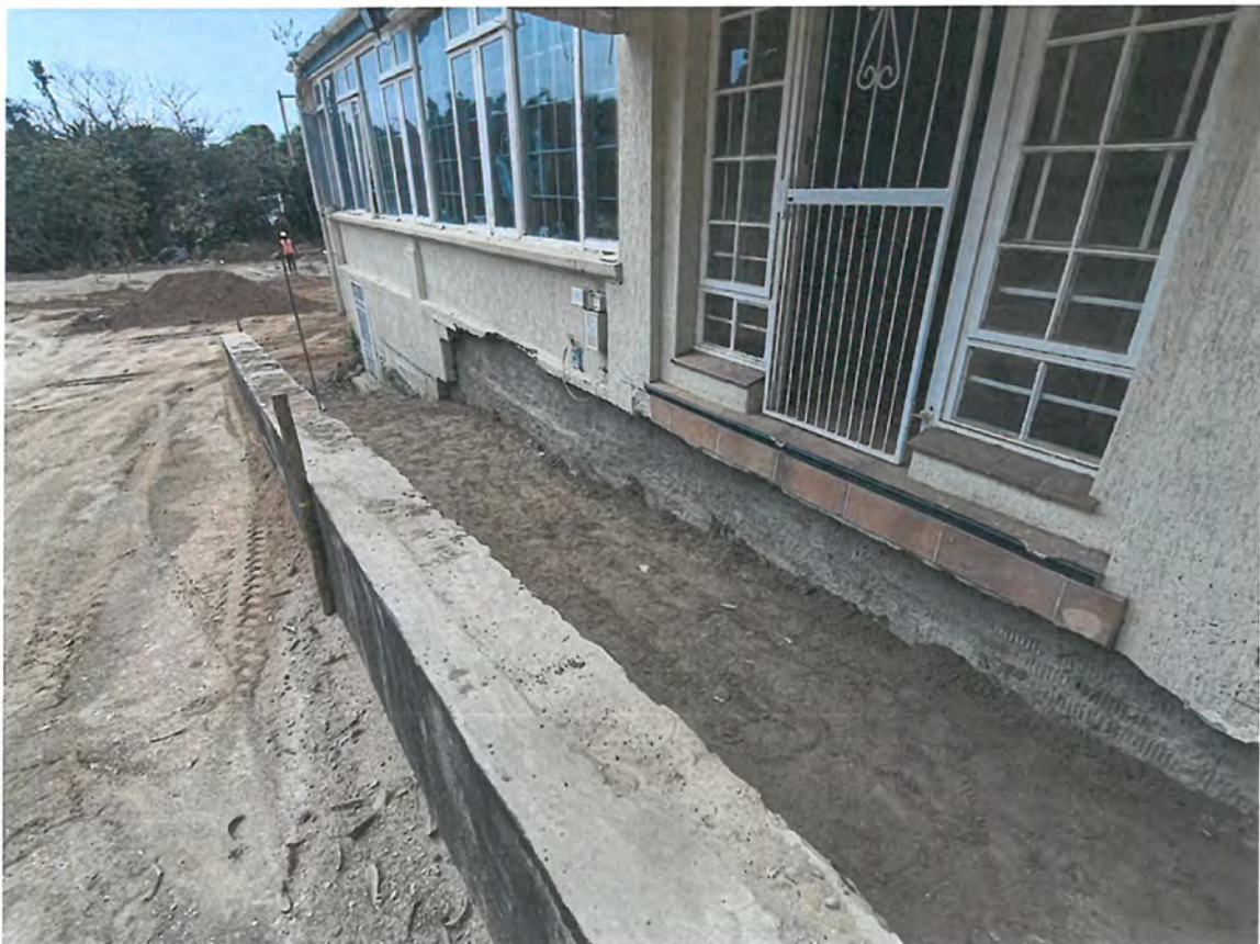
Repair work completed by 31 January 2022
