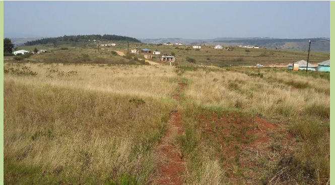
Plate 4: View of the disturbed pipeline's footprint near the Nkweletsheni reservoir. The P77 district road can be seen in the top right field of view.
