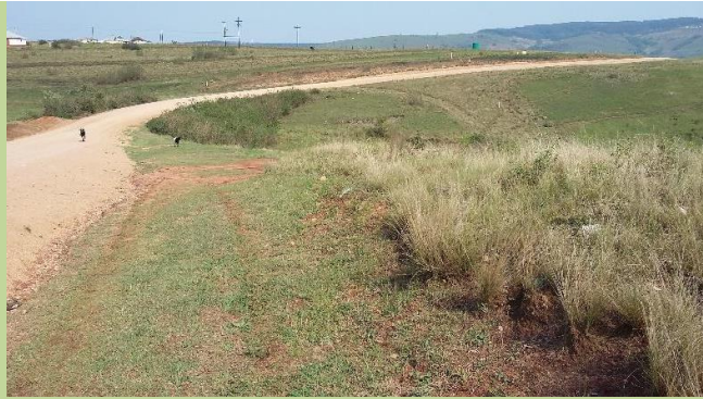
Plate 3: View of the disturbed pipeline's footprint near the Nkweletsheni reservoir. The P77 district road can be seen in the top right field of view.
