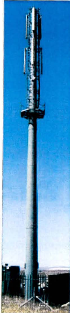
TYPICAL MONOPOLE MAST (PAINTED GREEN)
