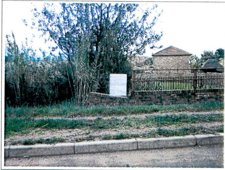
Site Notice 2 affixed at property boundary fence
