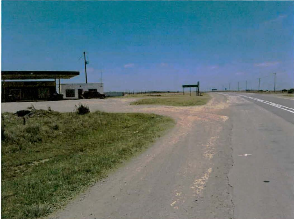
Figure 12: Fill Station along the N2.
