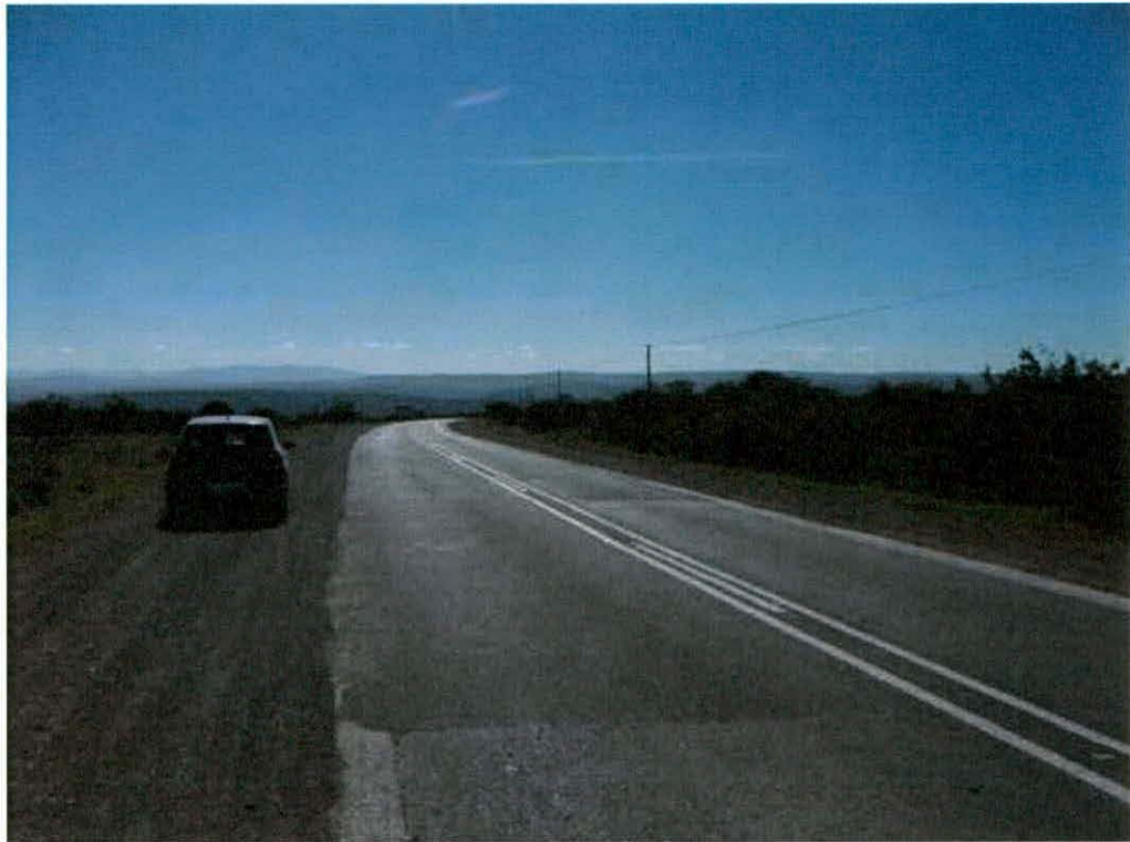
Figure 5: View of the Road
