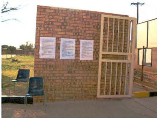
Ga-Seleka Hospital Gate
