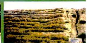
Spain - unstable and eroding highway fill treated with VS. Untreated eroded fill on right. VS grows well under low rainfall Mediterranean climate
