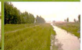
Vietnam - the left hand bank of the canal has been reshaped and stabilized with vetiver, the right bank has yet to be treated.
