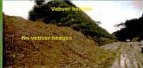
Vietnam - Ho Chi Minh Highway - with and without vetiver stabilization
