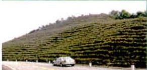
Vietnam: the Ho Chi Minh Highway has been stabilized with vetiver grass. The barriers and fills resist and withstand cyclonic rainfall events
