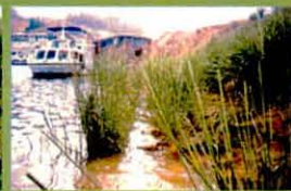
China - partially submerged vetiver grass used to stabilize the draw-down slope of a reservoir in Guangdong Province
