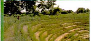
Congo D.R. - huge gullies that destroy urban areas and houses can be rehabilitated and stabilized using the Vetiver System.
