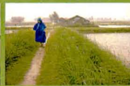
Vietnam - cyclone damage to sea dykes is a major problem. VS has been applied successfully for disaster mitigation
