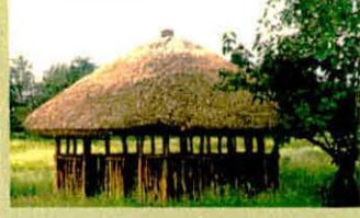
Zimbabwe - a nicely thatched meeting house using vetiver grass thatch. The thatch will last three times as many years due to its resistance to insects and fungus attack
