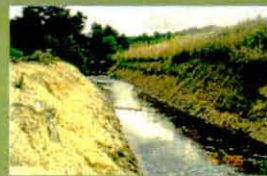
Australia - VS protects the right hand bank of a drain cut through acid sulphate soils of Queensland. Note left hand bank is devoid of any vegetation
