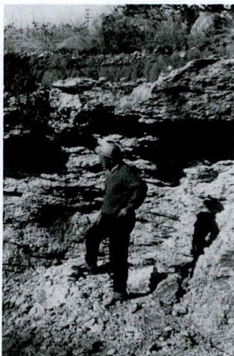
FIG. 1. Pseudobedded calcified alluvial sand (Netterberg 1980) with slight overlying hardpan development.
