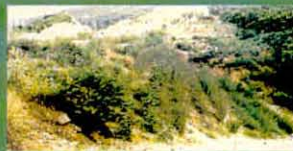
China - same fill less than a year later. After another two years this fill became fully forested. Untreated cut in background
