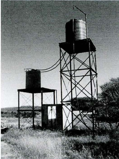
Figure 16: Storage tank for potable water
