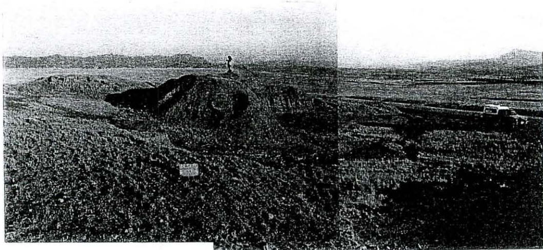
PHOTO 17: A north-westerly view of Borrow Pit 8036/3 at Stake Value km 13,1 (RHS).
