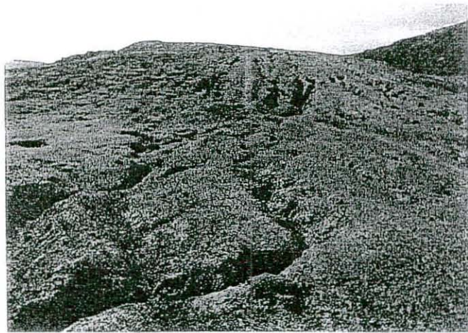
PHOTO 9: A view of the north-easterly part of Borrow Pit 715/3 at Stake Value km 9,7 (RHS), showing erosion scours in a rehabilitated slope.
