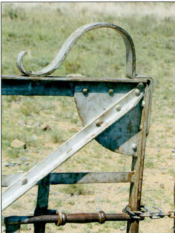
Fig.16 Detail of closing bolt of the fence gate, railway line on Knapdaar 14, Springfontein.
