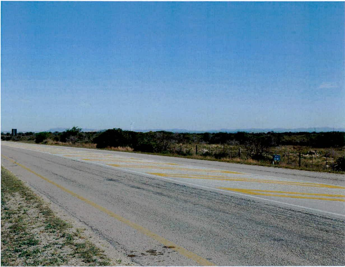
Figure 3.7 Photomontage of view from Photo Site 3 along the N2. The turbine is approximately 5km away.
