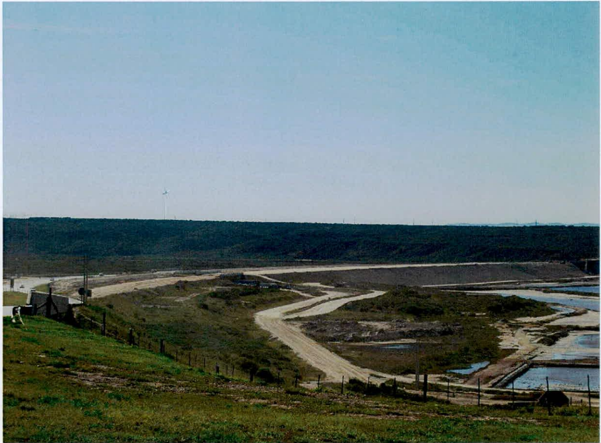
Figure 3.8 Photomontage of the view north from Photo Site 6. The wind turbine is a prominent feature on the terrace above the Coega River.
