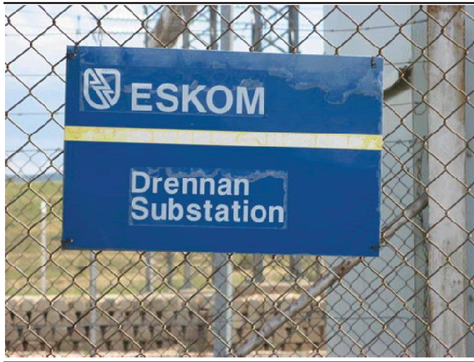
Figure 1.11 Existing Drennan Traction Substation Signage
