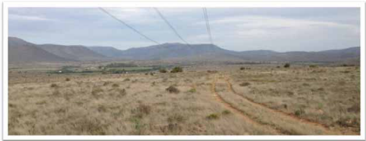
Photograph of Power Lines taken at Survey Point S5
