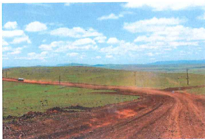
Photograph 2: Shows the upgraded existing track
