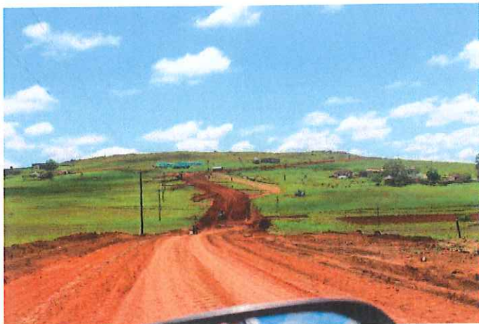
Photograph 1: Shows the upgraded existing track
