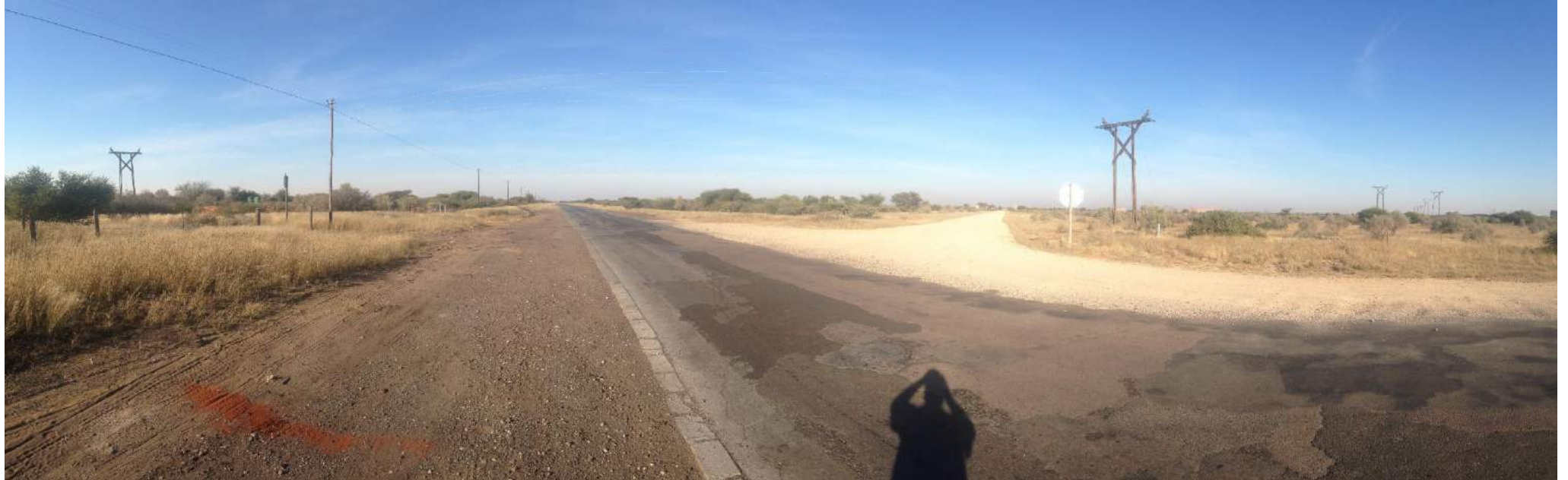
Photgrph looking south along the R380 to Deben. This is near to the location where the Umtu and Hotazel transmission line alternatives would cross the road.
