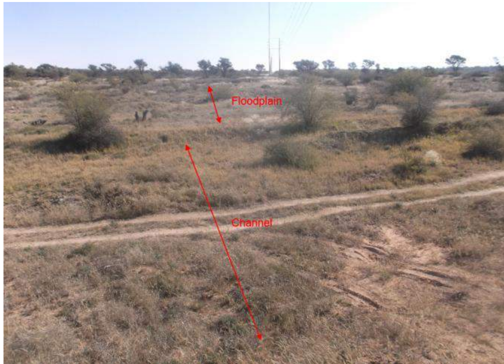
Figure 14 Existing transmission line crossing the Ga-Mogara River
