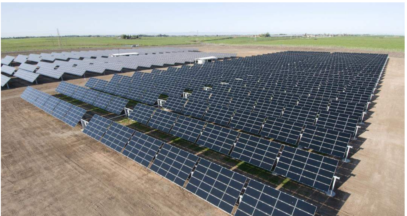
Figure 4: Photographic example of a Single Axis Tracking PV technology (Solar Professional)
