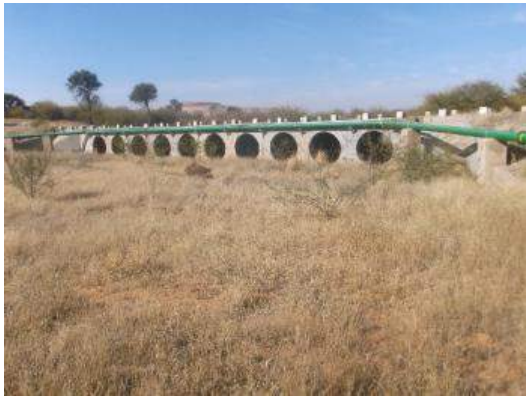
Figure 12 Road crossing of the Ga-Mogara River close to Eskom servitude
