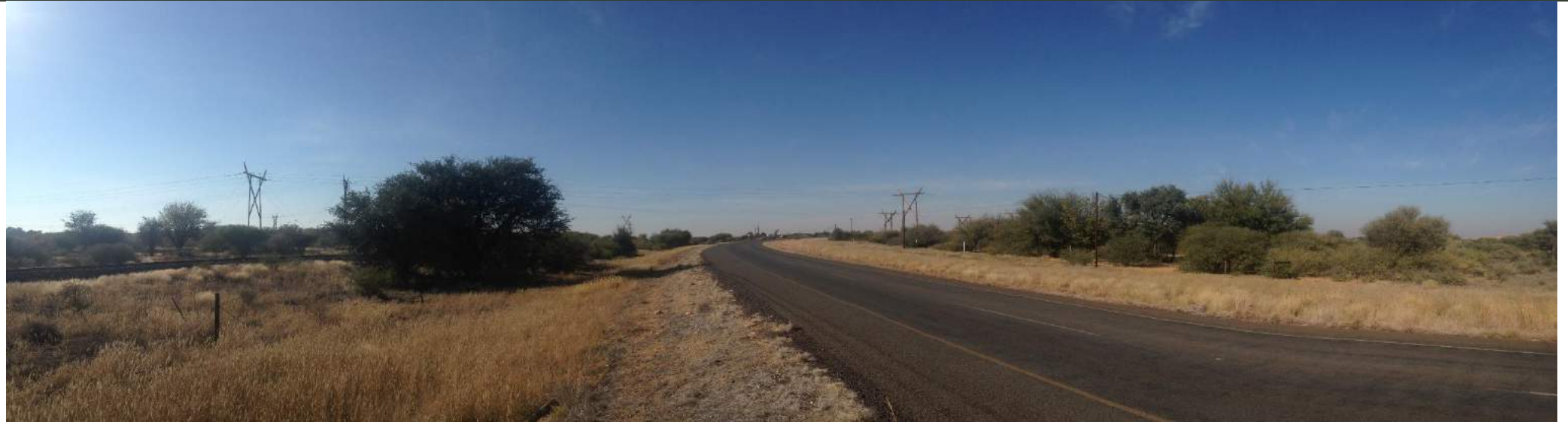
Where the Hotazel (Alternative 1) will cross the R31 close to Hotazel alongside other existing transmission lines
