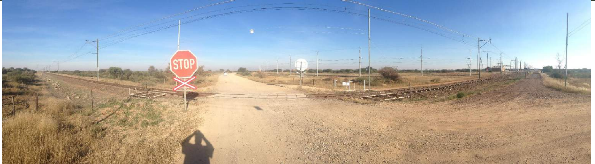
This is the main railway line into Hotazel. This location is approximately 1km north of where the Umtu and Hotazel Transmission lines would cross over the railway and associated electrical supplies, shown in picture.
