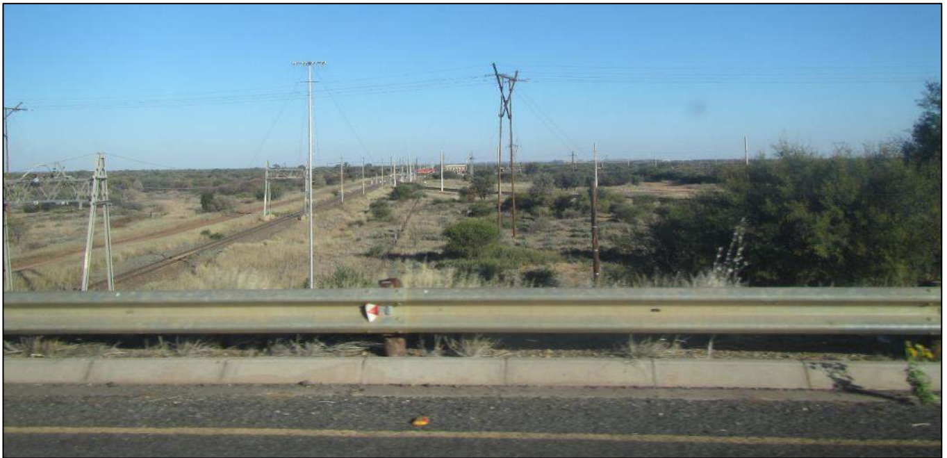
Figure 3: View towards the south from the road bridge over the railway showing infrastructure already present in the area.
